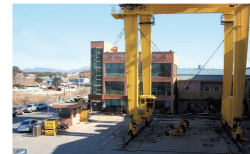
Site study for a design which fits the environment of the site exactly.
