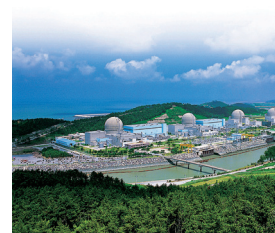
Emergency GenSets for Nuclear Power Plant
