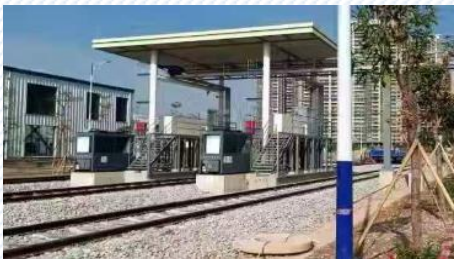
GaoMing HRS for Light Rail
